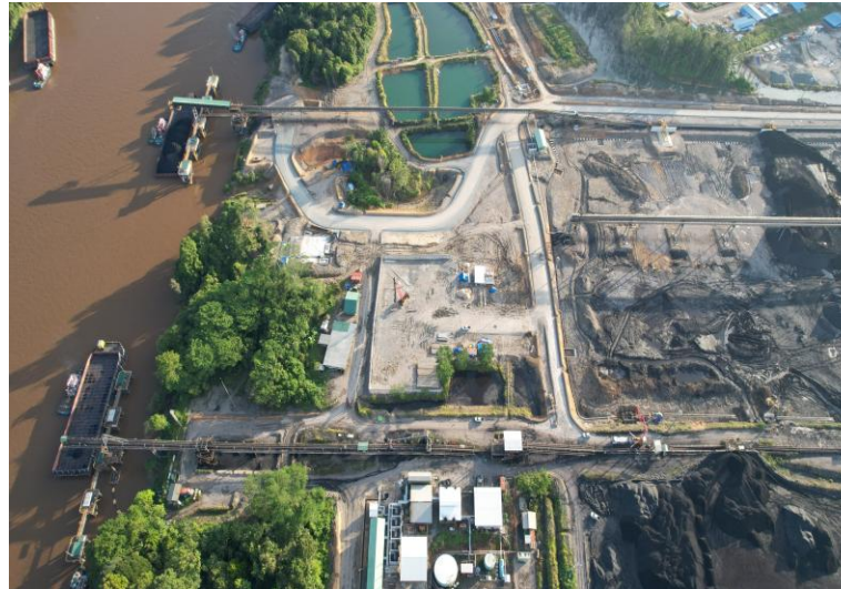
Second Barge Loading Conveyor
