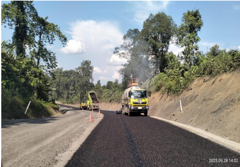
1 st phase of hauling road upgrade
